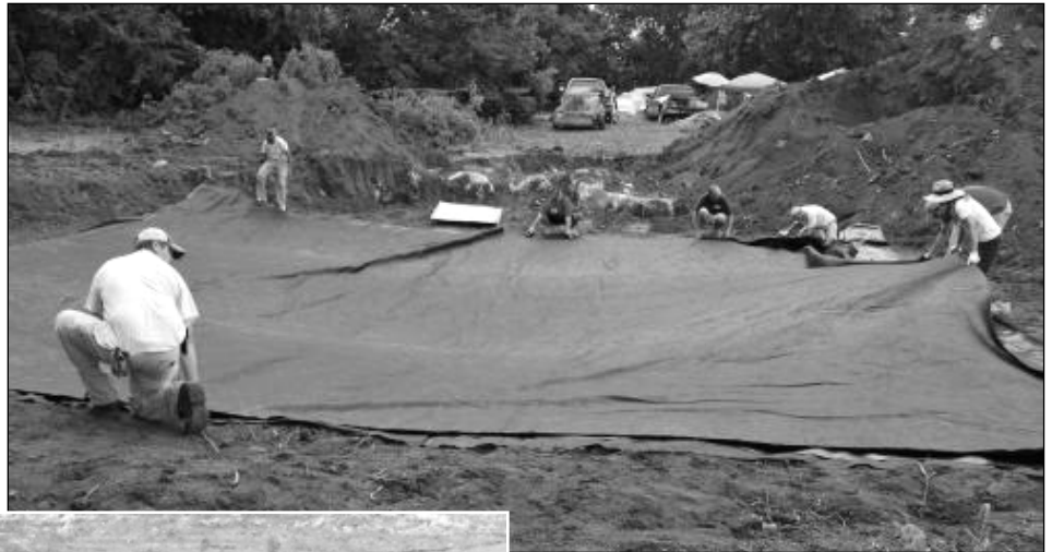
ABOVE: Volunteers install the liner for the vernal pond. LEFT: Bald cypress trees planted in the bio-retention basin.
