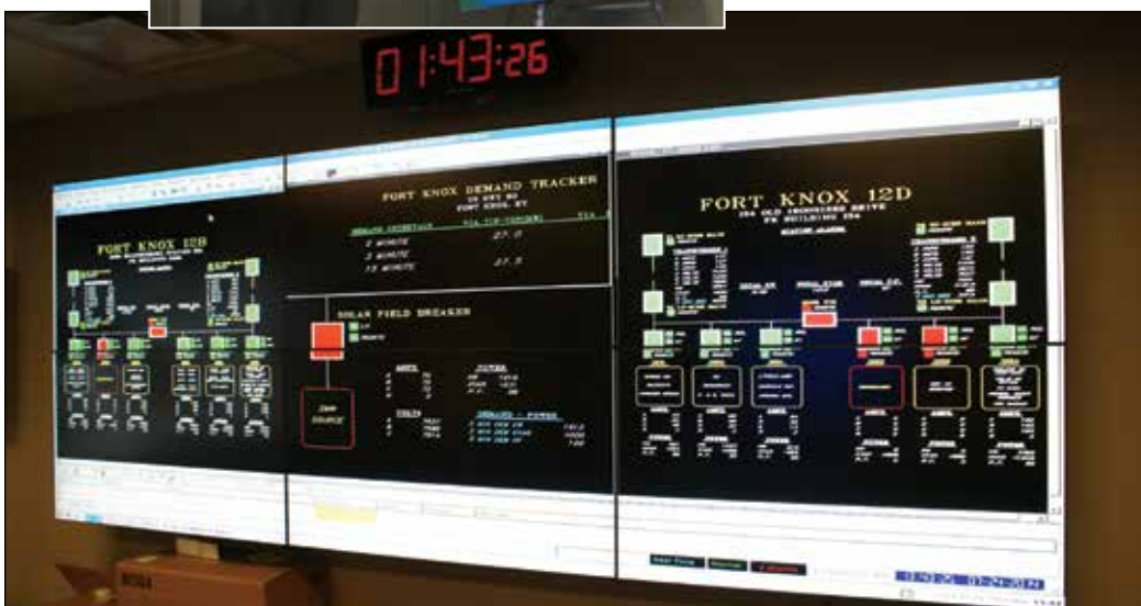
LEFT AND INSET: The Fort Knox monitoring system detects the energy levels in 300 individual buildings; Energy Manager R.J. Dyrdek. Photos by Tim Hughes
